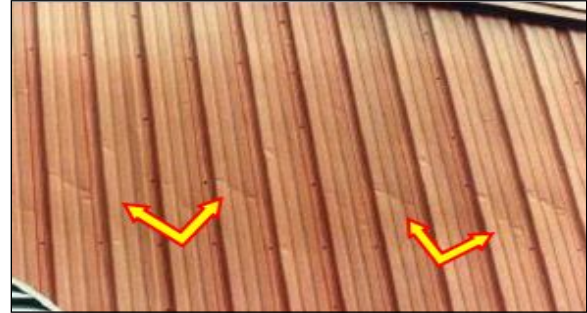
Figure 17-1 Carelessness During the Roof Installation Can Damage the Structure Siding
