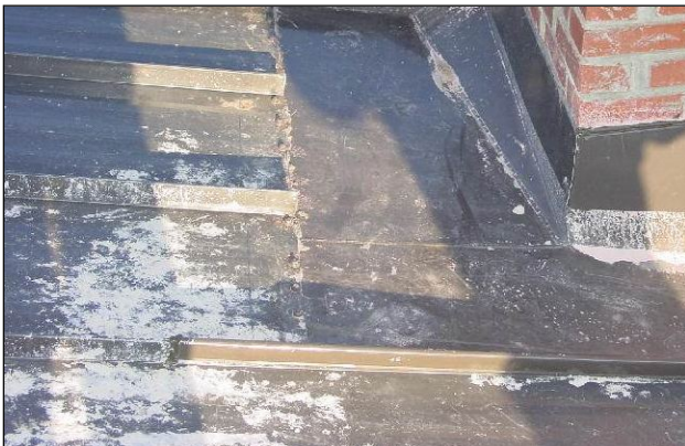
Figure 17-4 Mortar Droppings Should Be Cleaned Immediately.
