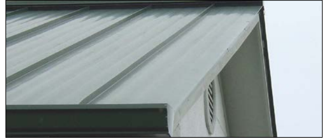
Figure 4-17 Architectural Panel Roof System
