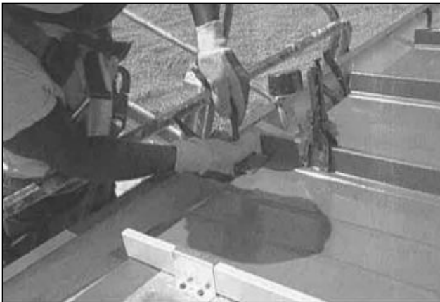
Figure 16-28 Spacer Tools Help Hold Panel Module
