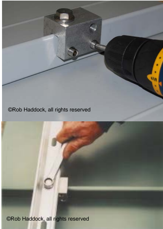
Figure 8-22 Example of Seam Mounted Fence System
