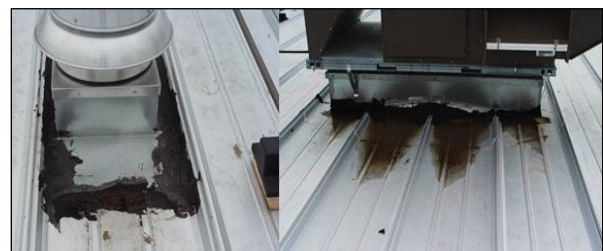
Figure 8-9 Improper Curb Types
