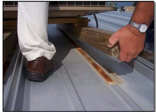
Figure 3-15 Roof Corrosion from Treated Wood
