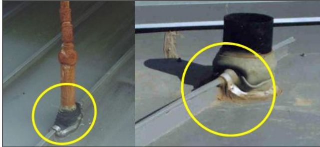
Figure 16-21 Poor Planning of Panel Installation Creates Areas Prone to Leak and Also Looks Bad
