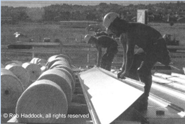
Figure 9-14 Proper Lifting Of a Roof Panel
