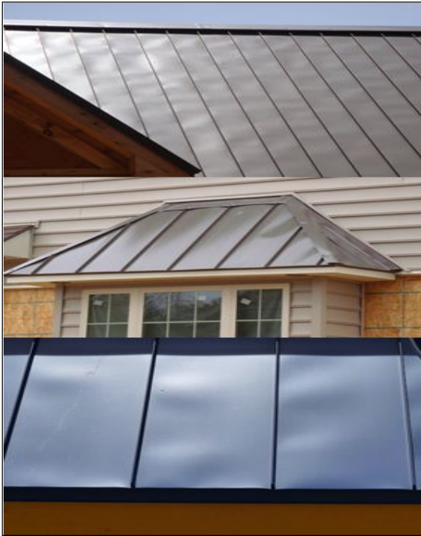
Figure 10-38 Oil Canning of a Metal Roof
