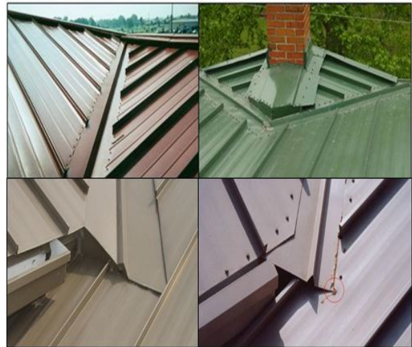
Figure 19-13 Valley Issues Affect Water Flow and Drainage
