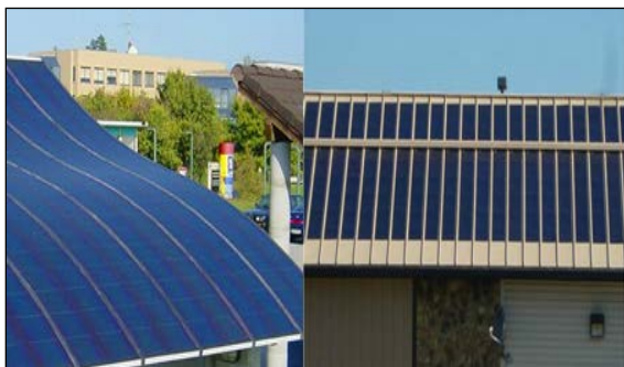
Figure 8-34 Photovoltaic Laminate on a Metal Roof
