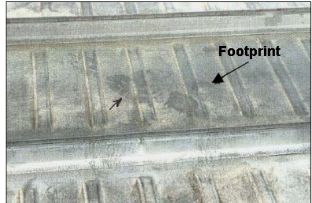
Figure 9-8 Inattention to Footwear May Cause Panel Damage
