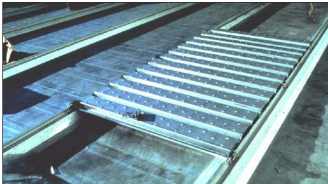
Figure 17-5 Installed Walkway for Heavy Traffic Areas
