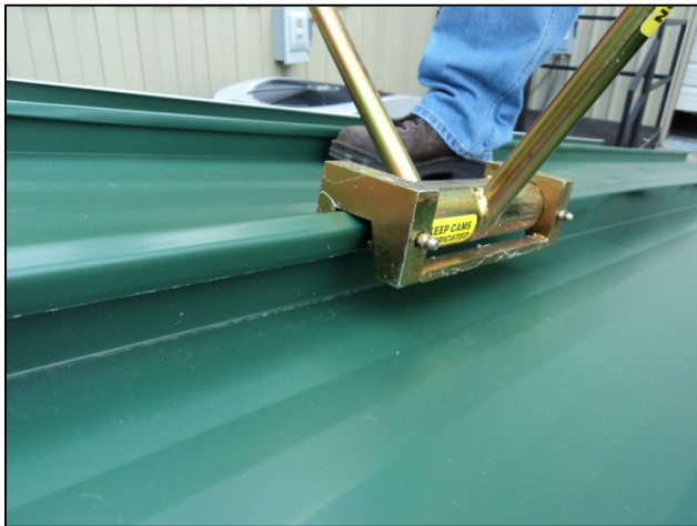
Figure 12-10 Hand-Seamer/Crimper
