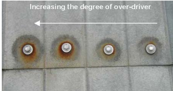
Figure 10-79 Over-Driven Fasteners
